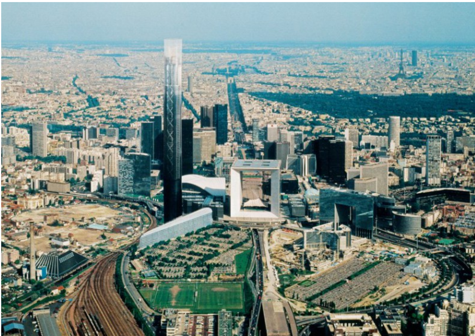
Our Same Fine, a project for building the world's narrowest skyscraper in line with Paris's historic Avenue des Champs-Élysées...
